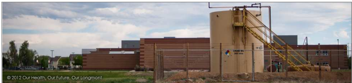
Natural gas well near school in Longmont Source: Our Longmont
