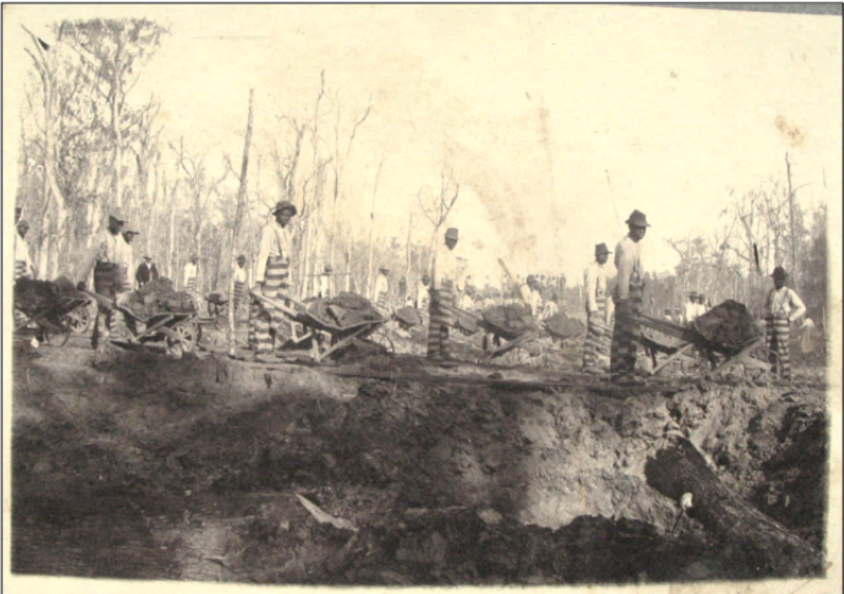
Figure 2.1. Leased convicts building a levee along the Atchafalaya River, Louisiana, 1901. (Source: Cardon 2017)
