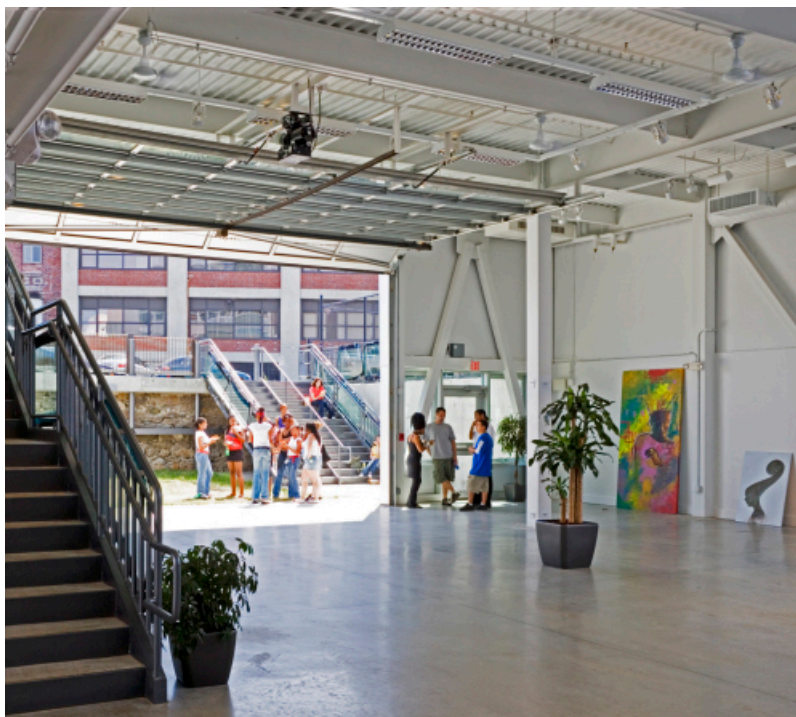
Figure 6.14: Large Opening Doors for Main Gallery – EpiCenter, Artists for Humanity
