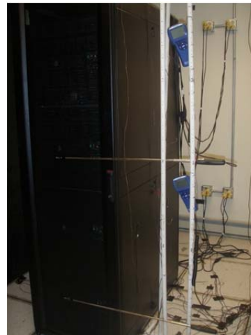
Figure 3–32: Anemometer Pole Set-up
