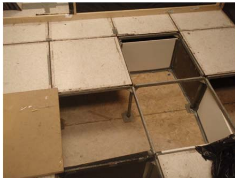
Figure 3–15: Raised Floor Plenum Partition Construction
