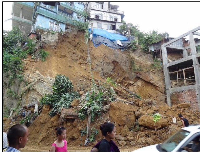
Figure 1. Landslide in Ramhlun neighborhood of Aizawl, June 2014 (photo credit: J. Rodgers).
