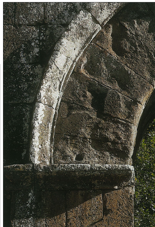
(b) Falerii Novi Arch Abutment
