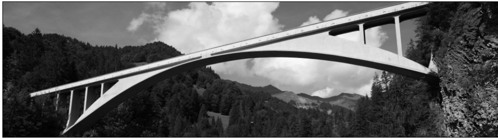
Figure 2.19: The Salginatobel Bridge, Schiers, Switzerland
