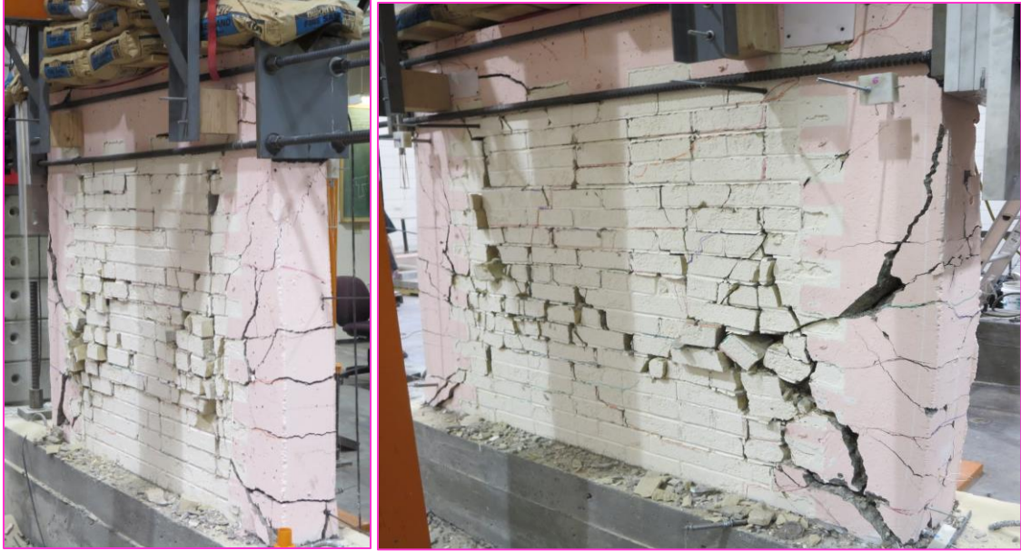
Figure 3-59. CM shear wall 1 failure mechanism
