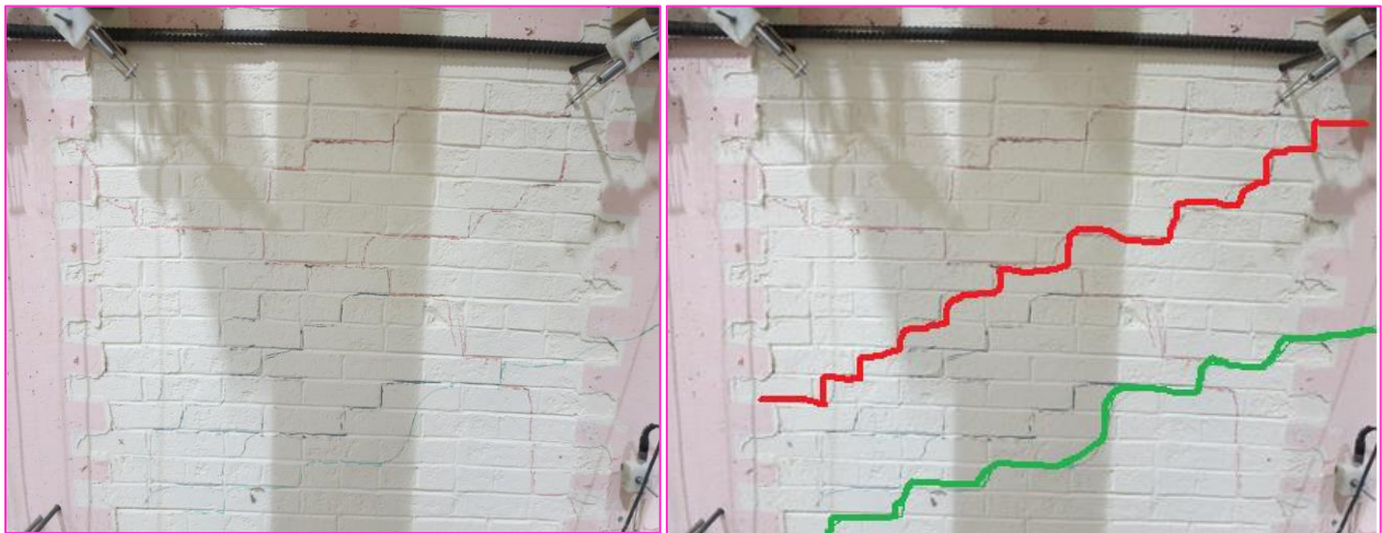
Figure 3-43. Nguyen CM Wall 1 shear cracks
