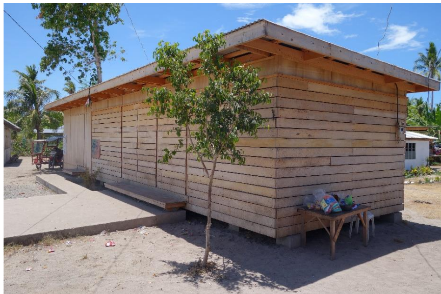
The completed community center provided additional space for social activities.
