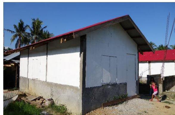
A completed core shelter after completion.
