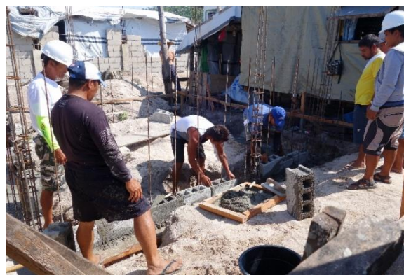
Demonstration training for block laying.
