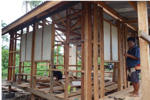
Construction of shelter walls.
