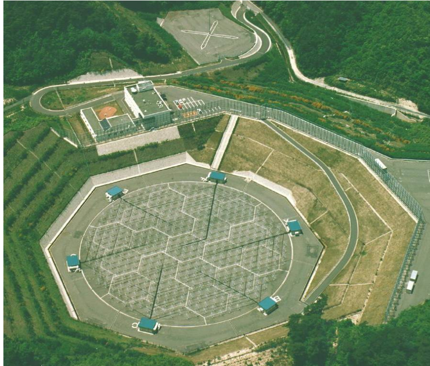
Figure 1.21. MU Radar in Japan. Built in 1984 and has a 103m overall diameter. Note the presence of an earth berm and metal fence for clutter reduction.
