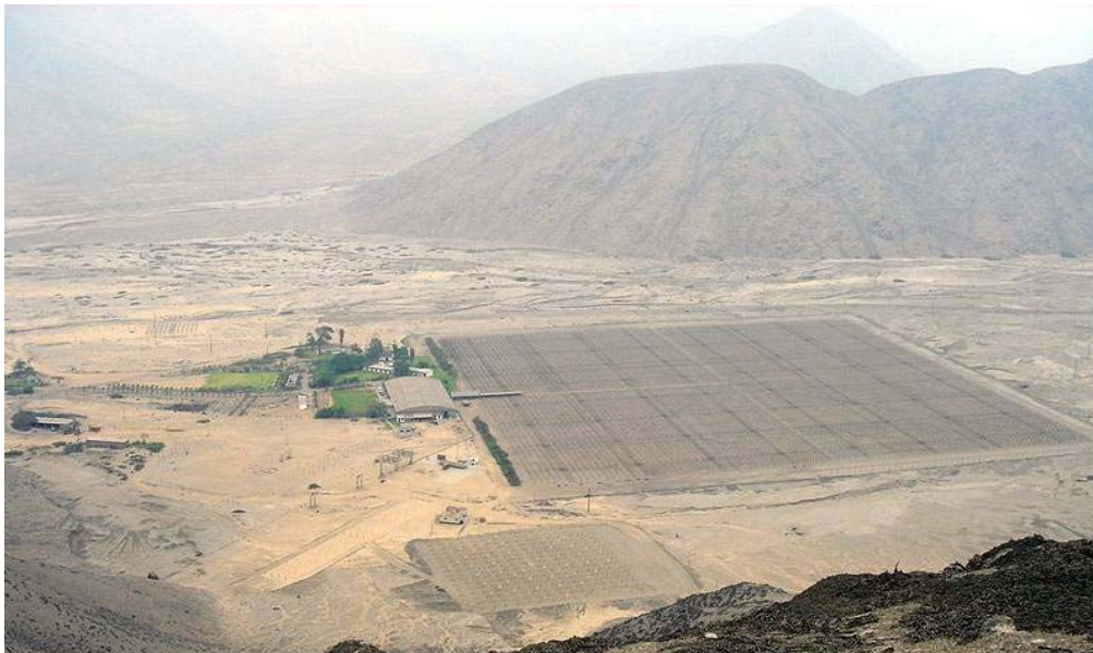
Figure 1.16. Jicamarca radar in Peru. The dimensions of the 18,432 element array are 288 x 288m [102].
