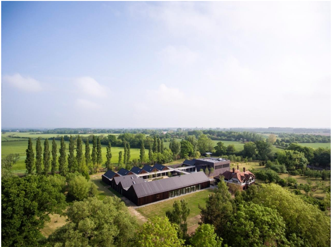
Figure 3.26 Vajrasana Retreat Centre, UK (Scott, 2016).
