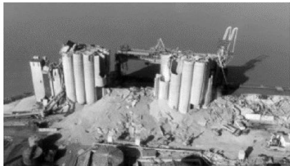
Figure 5 – View of the vertical silo after the accident
