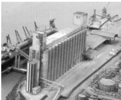
Figure 4 – View of the vertical silo before the accident (Masson, 1998)
