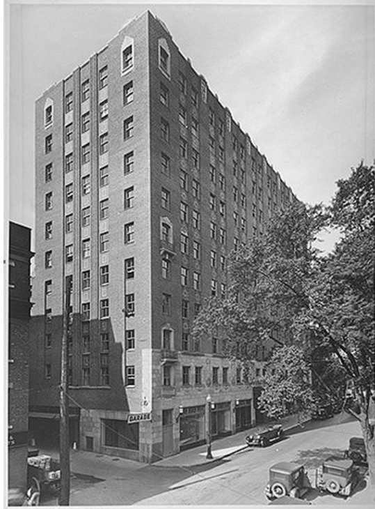
Figure 1. The Drummond Medical Building.
