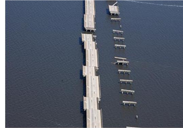
Collapse of I-10 Escambia bridge during Hurricane Ivan, Source: [4]
