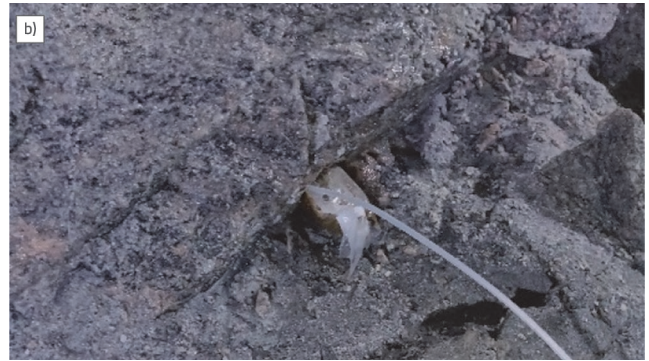
Figure 18. Water bags and site usage: b) Hole plugging with water–sand bags
