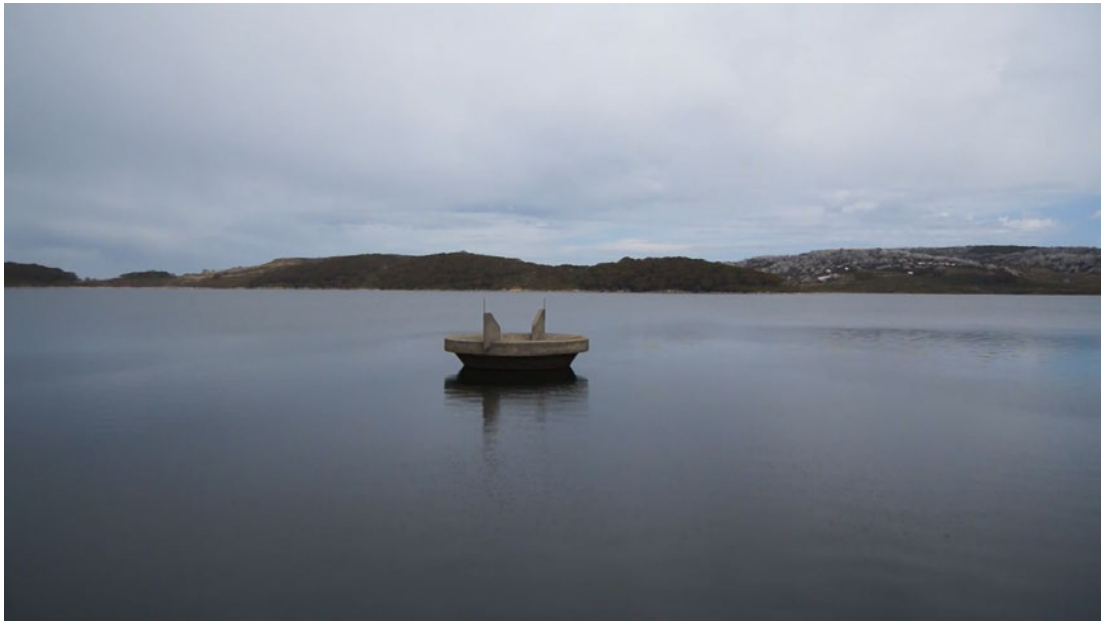
Rocky Valley Dam
