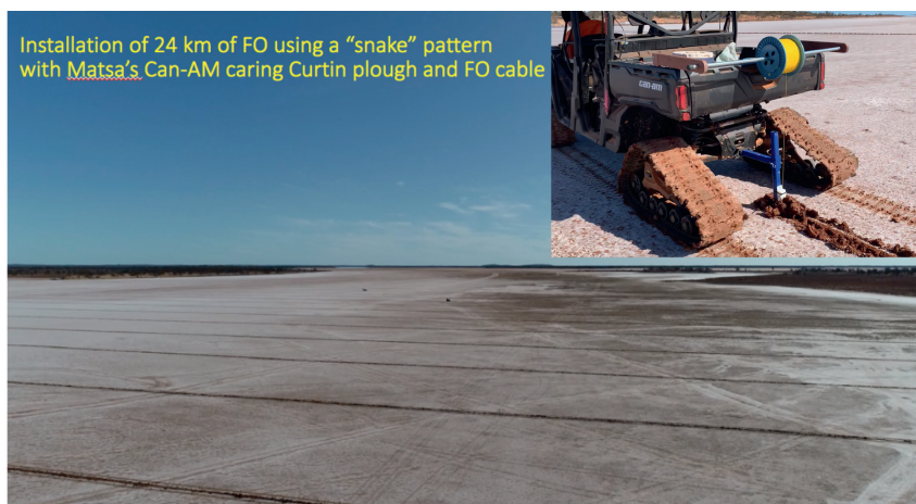
Figure 13 Curtin University designed and constructed cable plough attached to Can-Am 4WD vehicle. Provides very rapid deployment of FO cable approximately 0.1m beneath the lake surface. Some 24 km of cable was deployed in 10 h as a single man operation. This is equivalent of 32,000 sensors 0.8 m apart.
