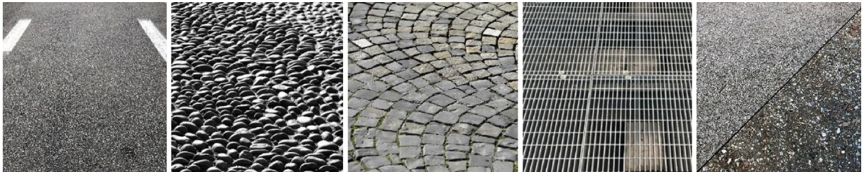
Fig. 3. Surface types, from left to right: bituminous conglomerate, uneven cobblestone, regular cobblestone, metal ventilation grid, and alternated dirt and concrete road.
