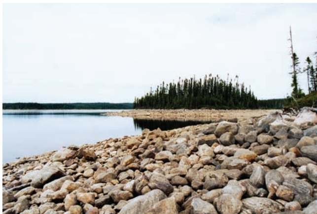
FIGURE 4. Wave-washed shoreline in thick (>2 m) till. A carapace of blocks and boulders has formed reducing further erosion of the shoreline; the large seasonal water level fluctuations of the reservoirs prevent the growth of lichens on the clasts, which facilitates identification and counting.
