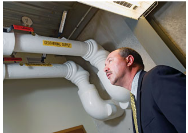
Bob Murray '82, dean of enrollment management, checks the center's geothermal system.
