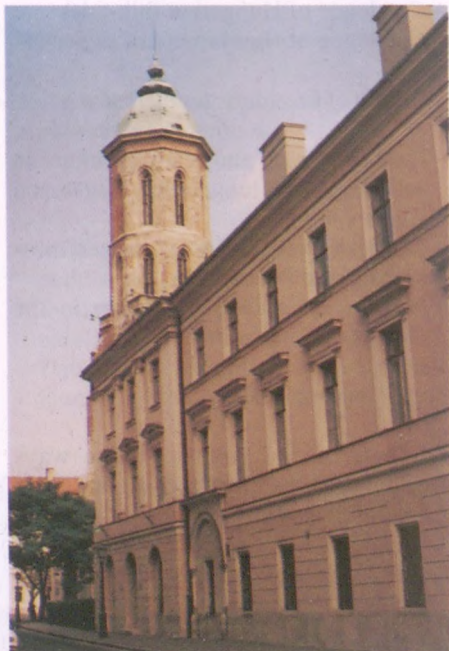
The main building of the institute
