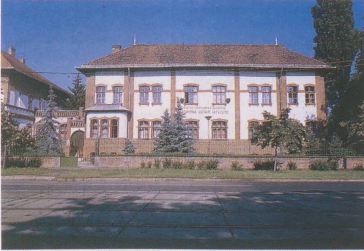
The main building of the institute
