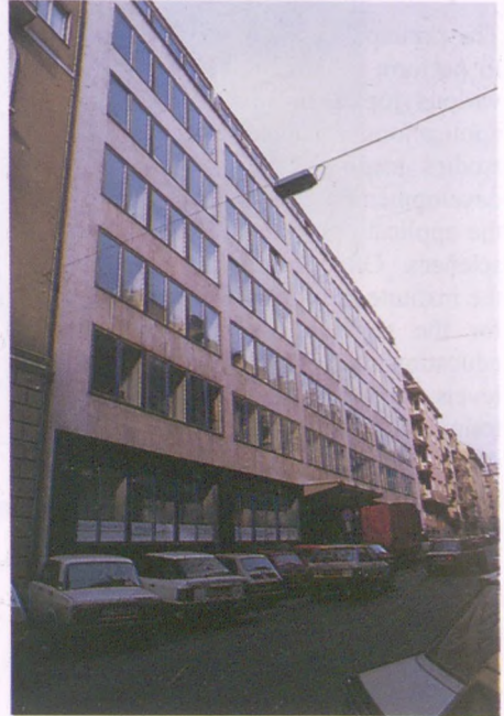
The main building of the institute
