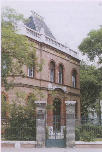
The main building of the Institute
