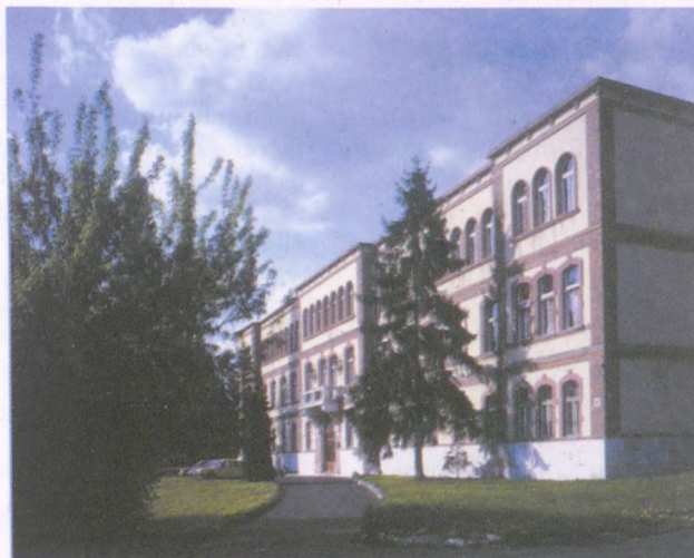
View of the main building of the research institute
