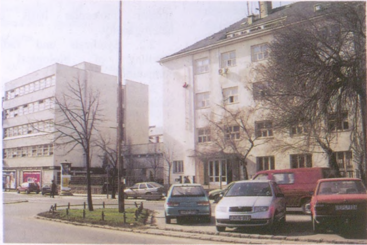
The main building of the institute
