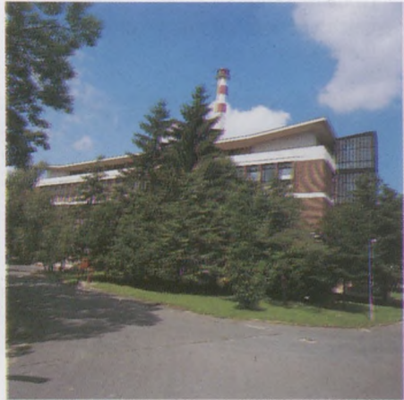
The main building of the research reactor
