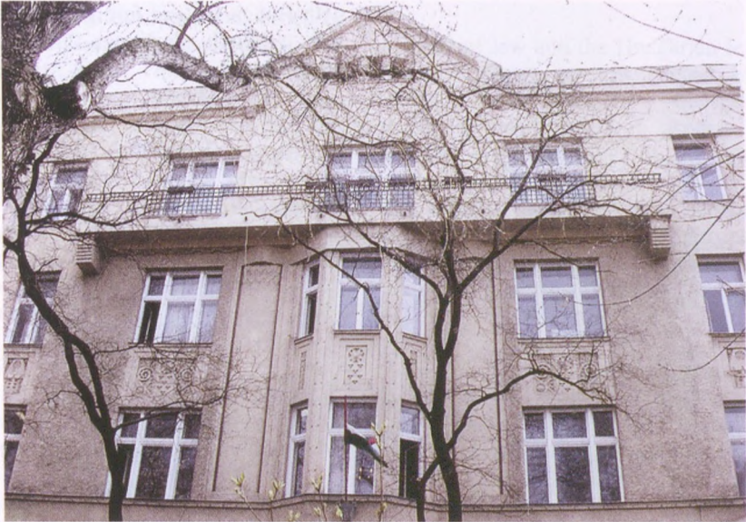
The main building of the institute
