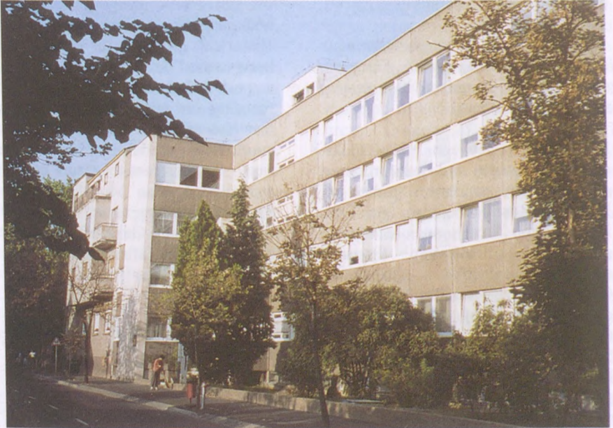
The main building of the Institute
