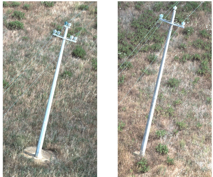
Fig. 1: An example of a difficult pair taken from the dataset: the two poles have a very similar structure and are set against similar background. However, they can be distinguished by carefully looking at their assets (in particular, their isolators).
