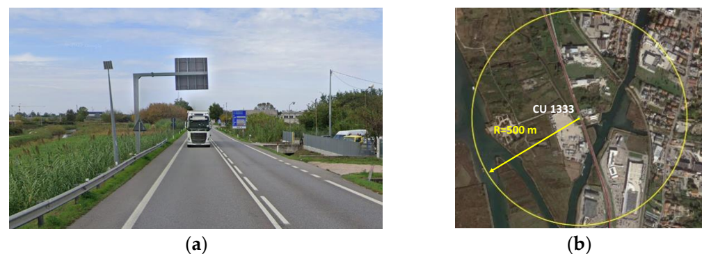
Figure 4. Control unit 1333 on the national road n.309: (a) installation site with two lanes; (b) surrounding 500 m radius area (Google Earth).
