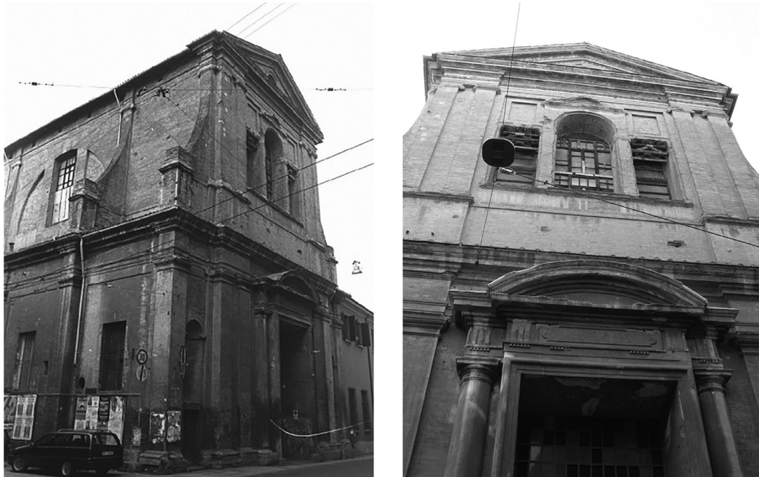
Fig. 2. The former Church of San Barbaziano. Source: https://www.beniculturali.it/ .
