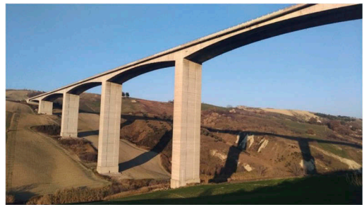
Figure 1. Sud-Est view of the Bridge.
