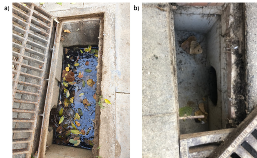
Figure 2. Sand sewer with accumulated water before the modification (a) and modified sand sewer with its bottom filled with concrete to the level of the base of the discharge pipe (b).
