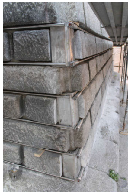
Figure 7. Post tensioned steel bars (B).
