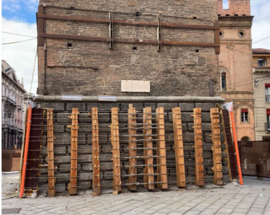
Figure 6. Confinement of the bugnato (C).
