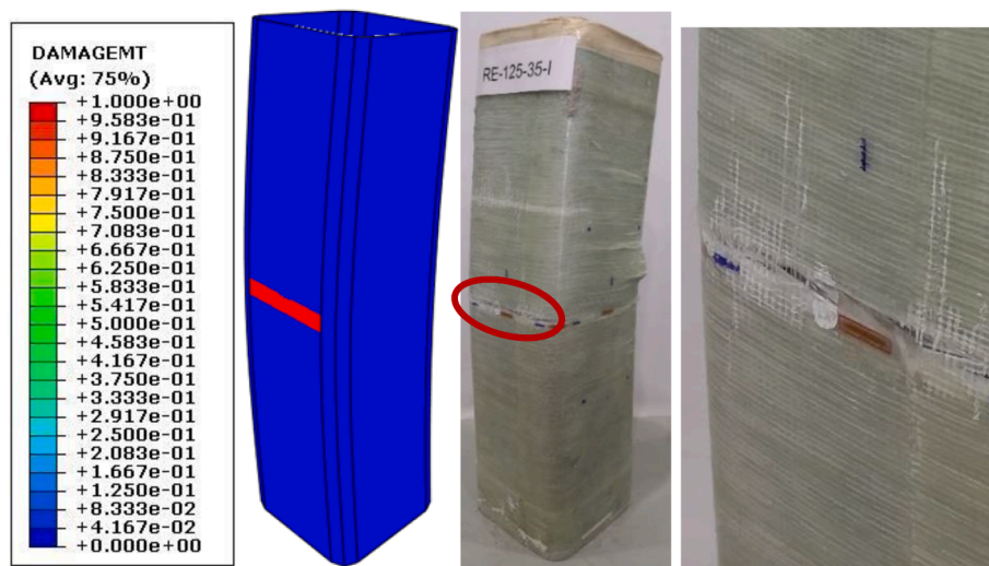
(b) GFRP matrix failure on the tensile side
