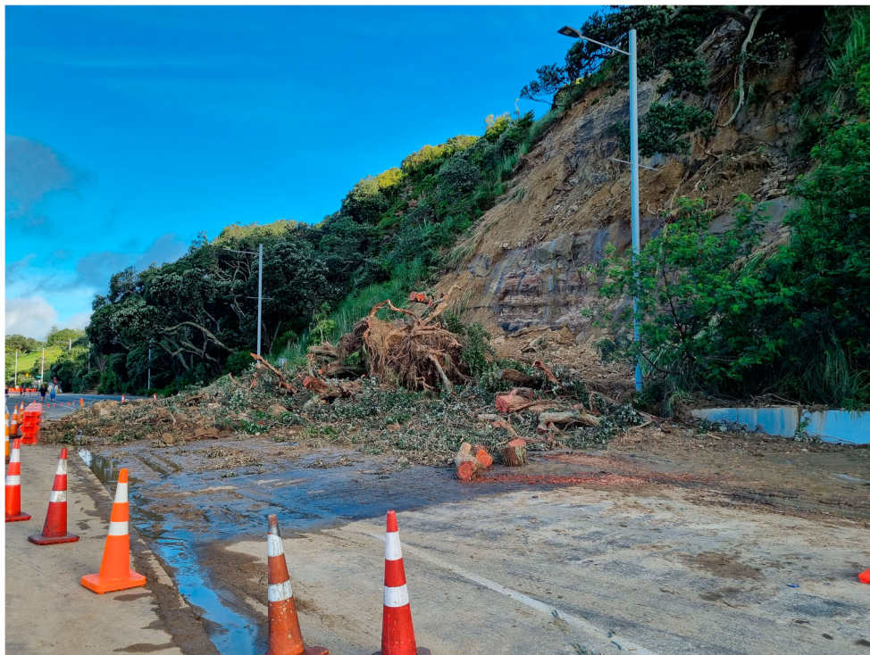
Figure 3. Tamaki Drive land slip after the extreme rainfall event on 27th January 2023. In this photograph, a large tree that fell onto the road had already been partially cleared. This is a major road serving the eastern bays of Auckland and it remained closed for several days.
