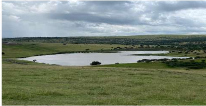
Observation data: Mxumbu dam used for irrigation and for livestock watering
