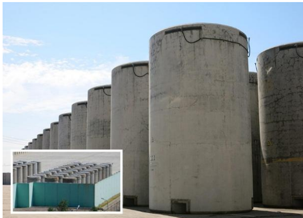
Fig. 1. Storage containers of Zaporizhska NPP
