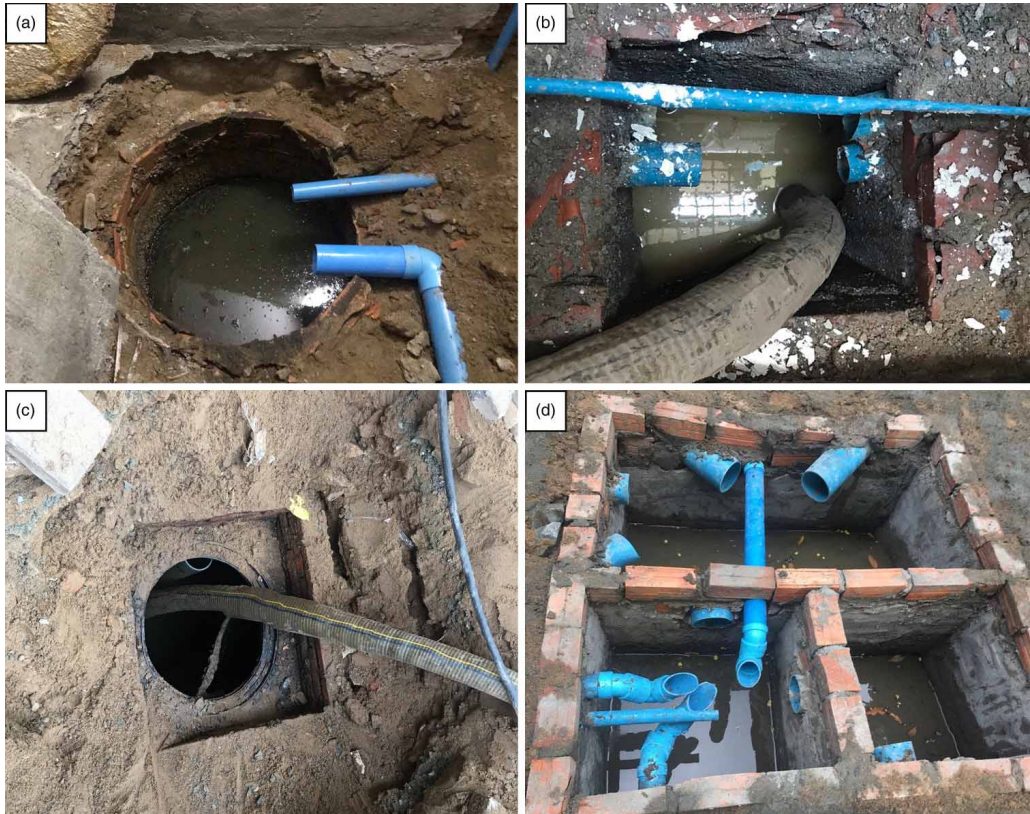
Figure 1 | Typical (a) circular and (b) rectangular cesspits and (c) imported plastic and (d) rectangular brick septic tanks used by households in Phnom Penh. Please refer to the online version of this paper to see this figure in colour: http://dx.doi.org/10.2166/washdev.2021.193 .
