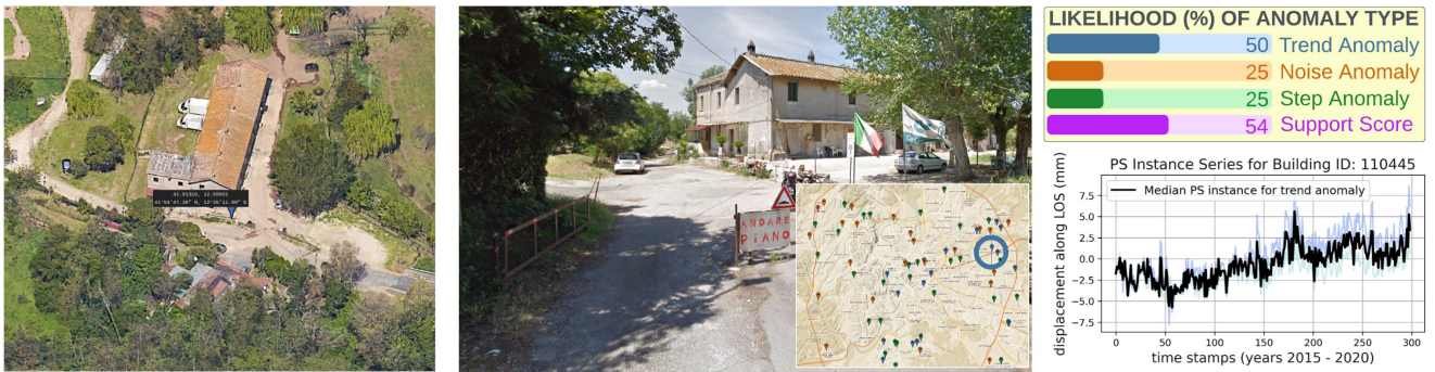
Fig. 15. Farm house with the detected anomaly of trend . Upon inspection of both aerial and street views, it was observed that the building is old and poorly maintained, which could possibly account for the detected displacement.
