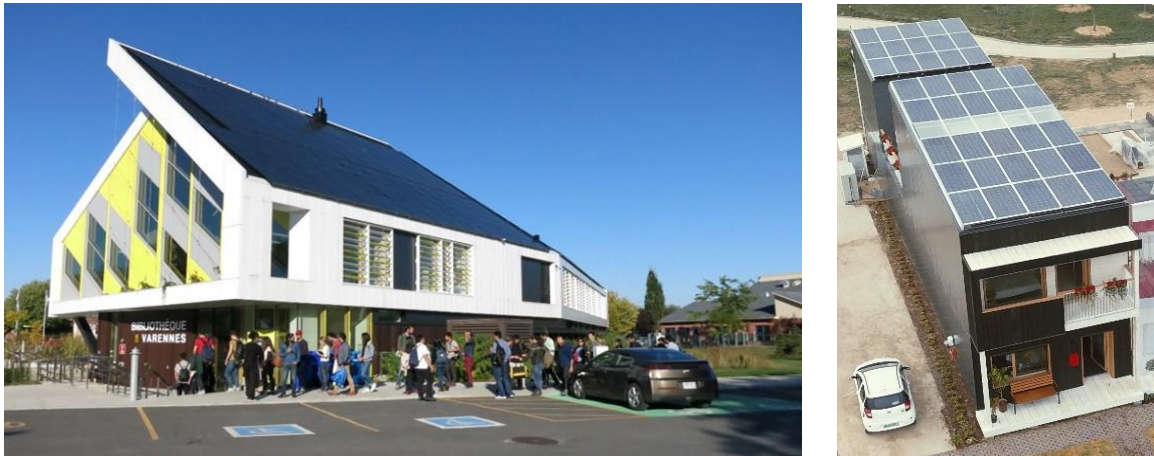
Figure 1-4 The Varennes Library (left), the first institutional Net-Zero Energy Building in Canada and the Team Montreal Deep-Performance Dwelling from the Solar Decathlon Competition 2018 in China (right), with BIPV/T.
