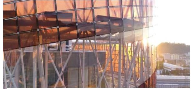
Figure 0-11 Science Tower, Graz, Austria. Innovative glass of 3mm thickness by H. Glass
