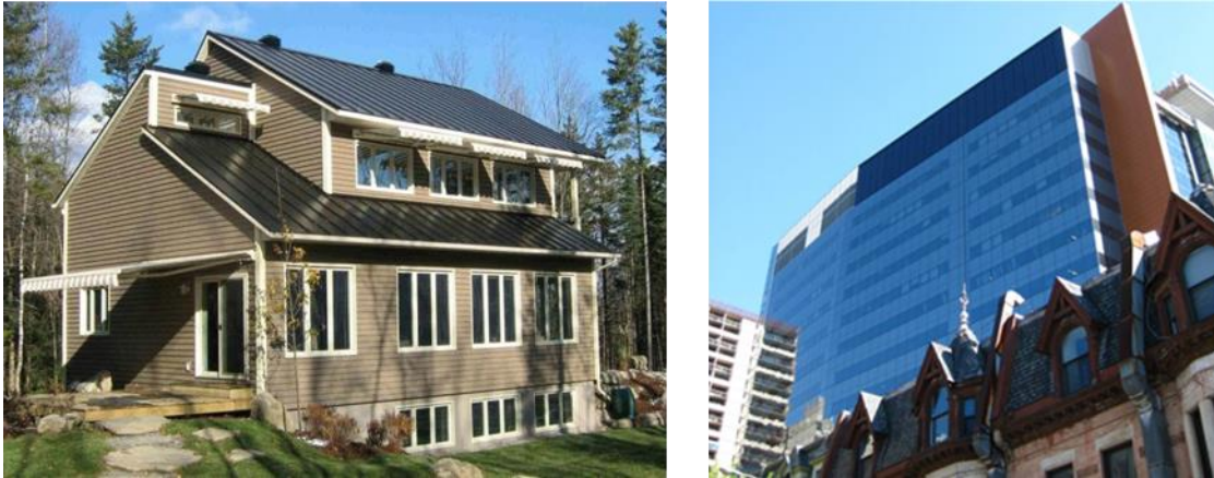
Figure 1-3 Both Eco-Terra house (Left) and JMSB building, have BIPV/T (right)
