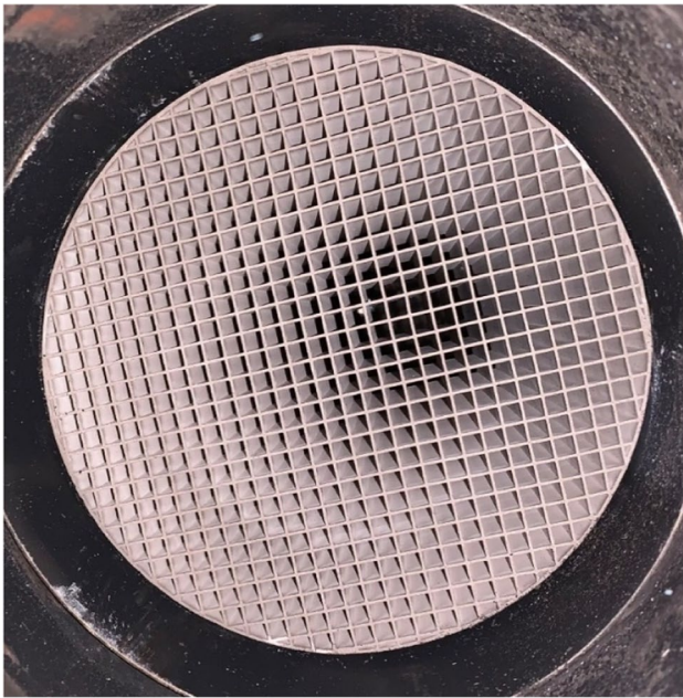
Fig. 2 Tested catalyst installed into the flue gas duct
