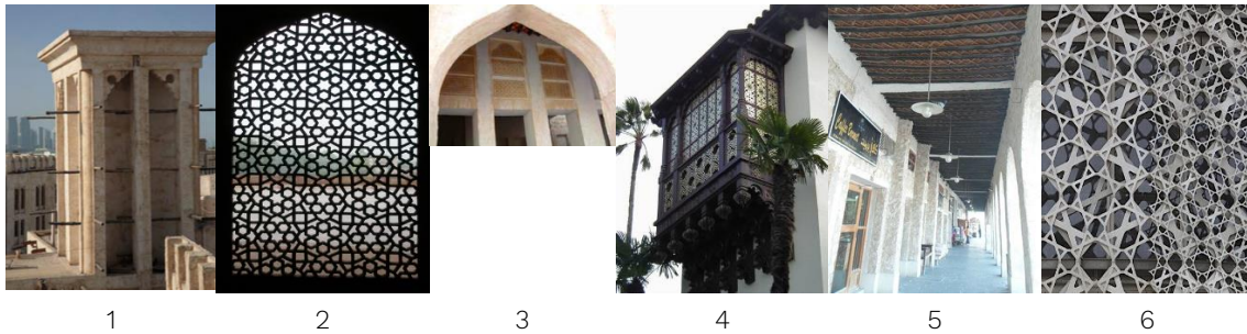
Figure 13. The selected elements for the assessment (1.Barjeel/wind catcher, 2.Screen with Islamic pattern, 3.Pointed arch, 4.Mashrabiya, 5.The traditional wooden roof, 6. Modern Islamic pattern)
