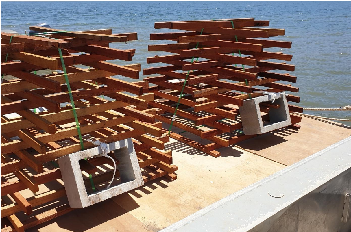
Figure 7 Timber cribs assembled on the deployment pontoon
