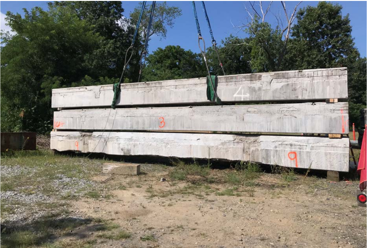
Figure 4.9: Essex Bridge beams at the Brack Structural Engineering Laboratory (UMass Amherst)
