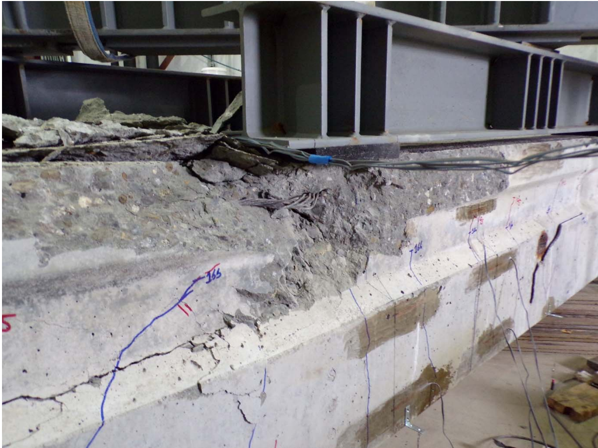
Figure 5.13: Concrete crushing at failure of Specimen R3
