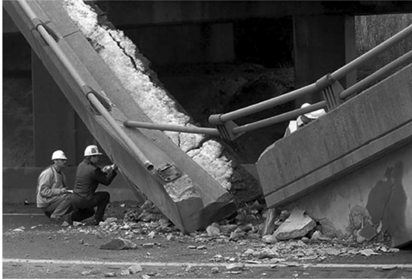
Figure 2.1: Lake View Bridge collapse
