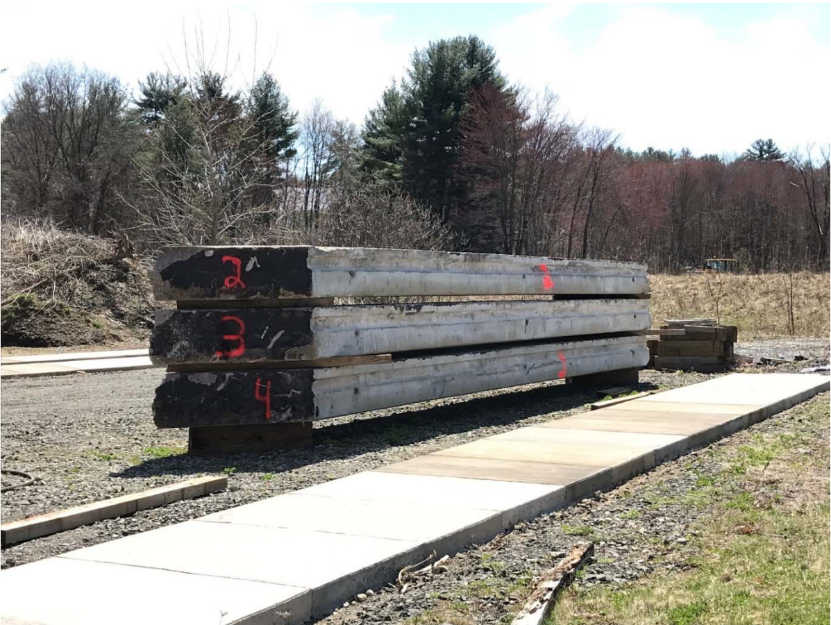
Figure 4.6: Rehoboth Bridge beams at Brack Structural Engineering Laboratory (UMass Amherst)
