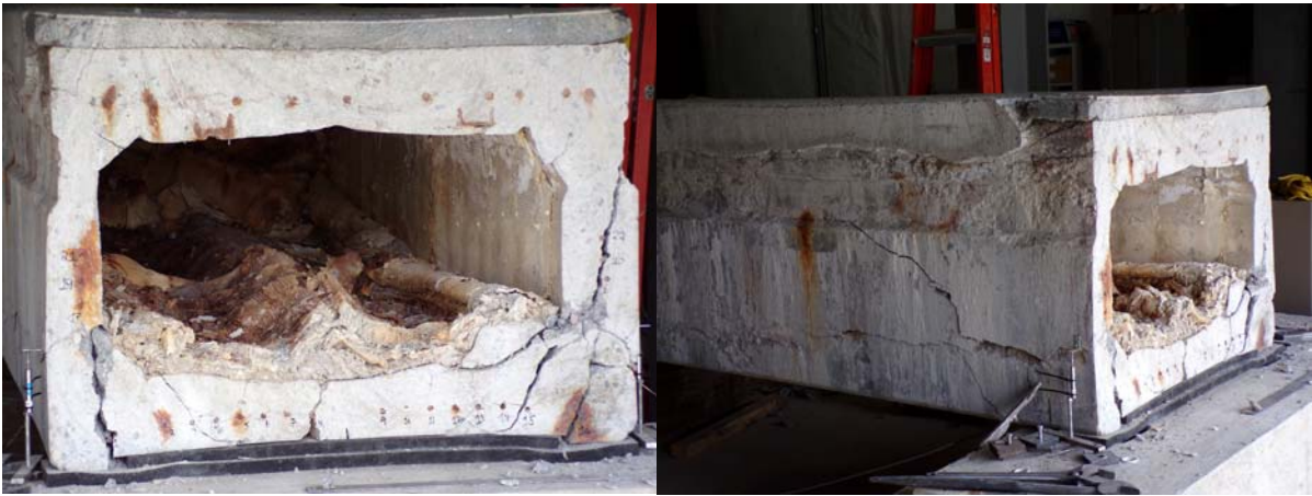
Figure 5.22: South end failure of Specimen E4
