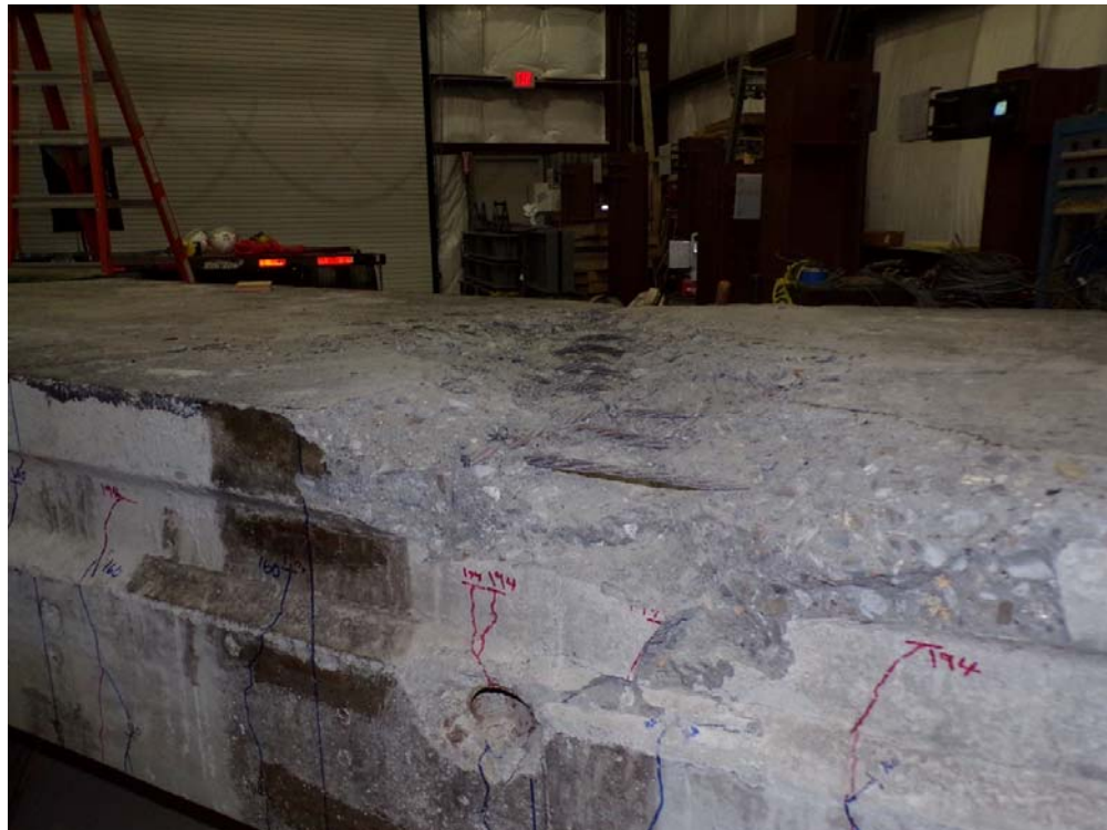
Figure 5.17: Concrete crushing after failure of Specimen R4
