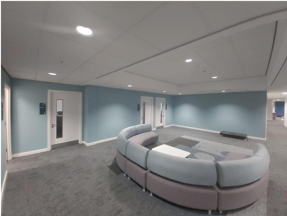
Figure 5.12: Waiting Space, Academic staff offices with Surface IP64 Led Circular Dimmable Luminaire C/W Polycarbonate Diffuser Lighting fixtures (Percy Shaw House Building).
