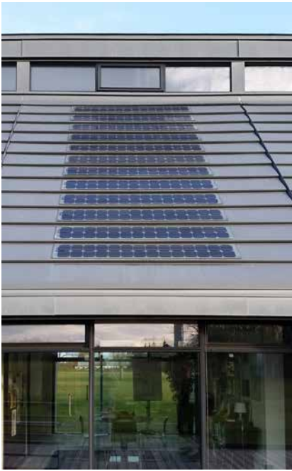
FIG. 4.6 Building Integrated Photovoltaics (BIPV) or other means of energy generation is needed to create buildings that are almost energy neutral. Balancing energy demand and generation is difficult because it depends on buildings and installations but also on the type of use, comfort demand, and user behaviour. The architectural integration of components is a future challenge for designers. (Image by the author)
