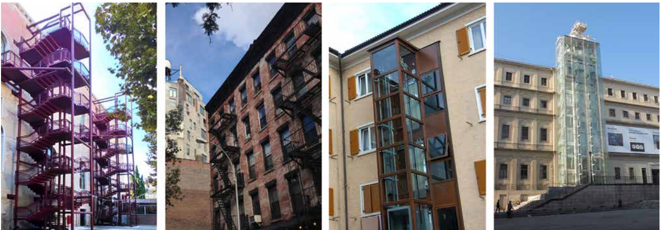
FIG. 3.2 Examples of functional additions for accessibility and security: architectural prosthesis. From left: security stairwell in a historical building, Tolentini, Venice; external security stairs in New York (Image by Lidia Savioli, 2015); external lift in Bolzano (Image by Comune di Bolzano, 2014); external lift in the Reina Sofia Museum, Madrid (Image by Valeria Tatano, 2014)
