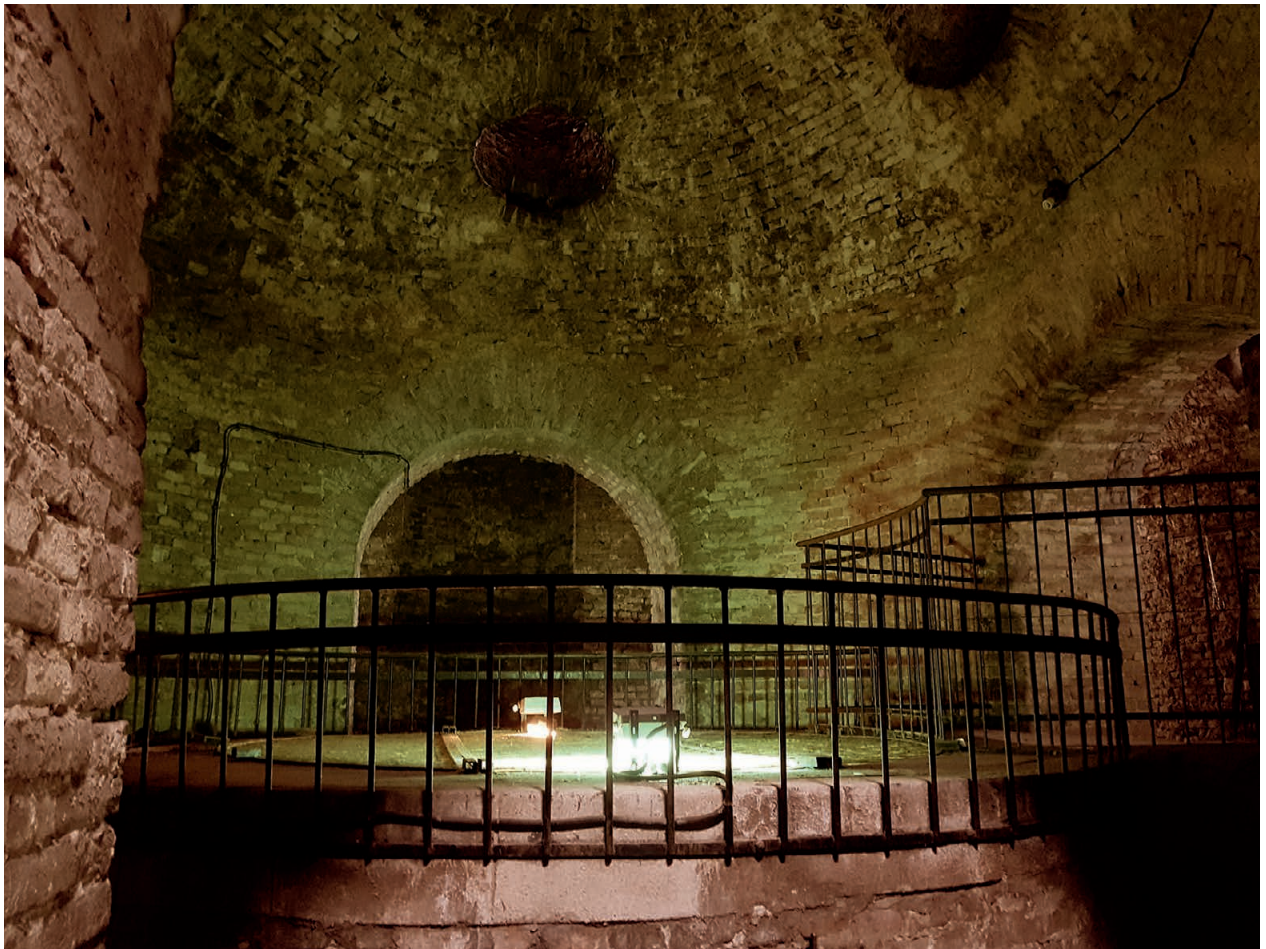
Fig. 56. Great Well in the Belgrade Fortress – working platform over the dry shaft in the protective entrance structure (PE Belgrade Fortress)
