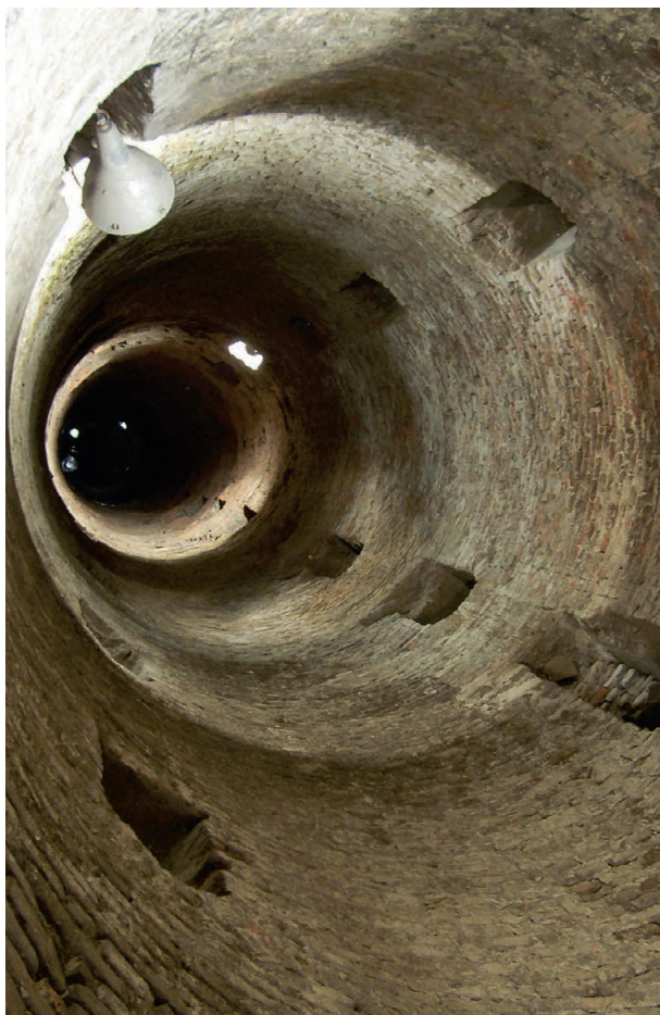
Fig. 57, 58. Great Well – the dry shaft and spiral stair flight (PE Belgrade Fortress)
