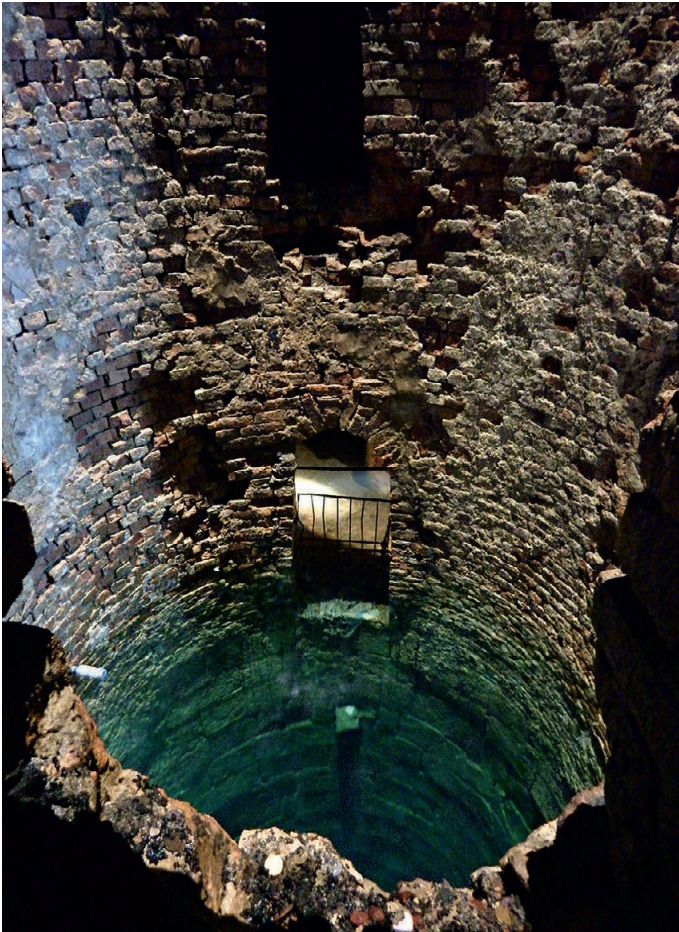
Fig. 59. Submerged well shaft serving as a cistern (PE Belgrade Fortress)
