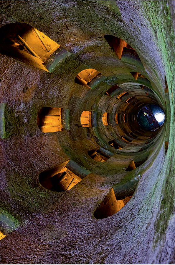
Fig. 53. Fortress well in Orvieto – view towards the water at the bottom of the dry shaft surrounded by spiral staircases
