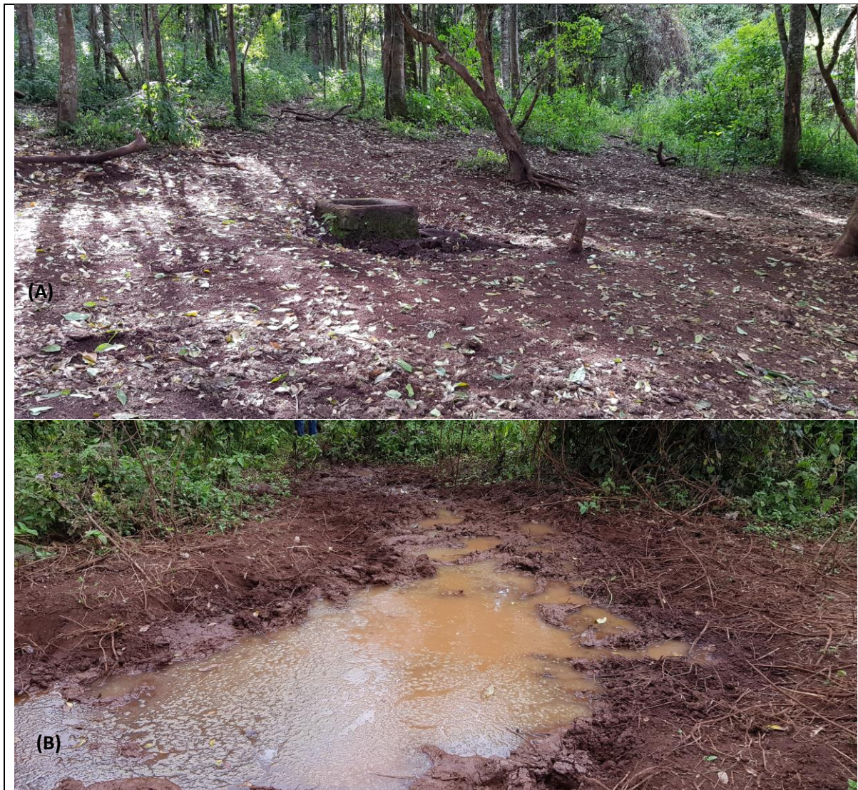
Figure 4. 13: (A) Bare land around an open water chamber due to trampling and (B) leakage of a water pipe broken by wild animals searching for water in KINAPA.
