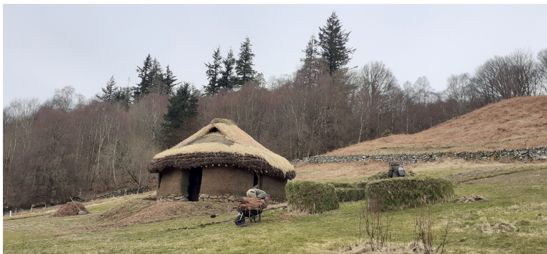
Figure 7: The modern turf structures built at Comrie Croft, Perthshire, central Scotland; left: roundhouse structure with modern windows and stove; right: turf bench. Photographs: Tanja Romankiewicz.
