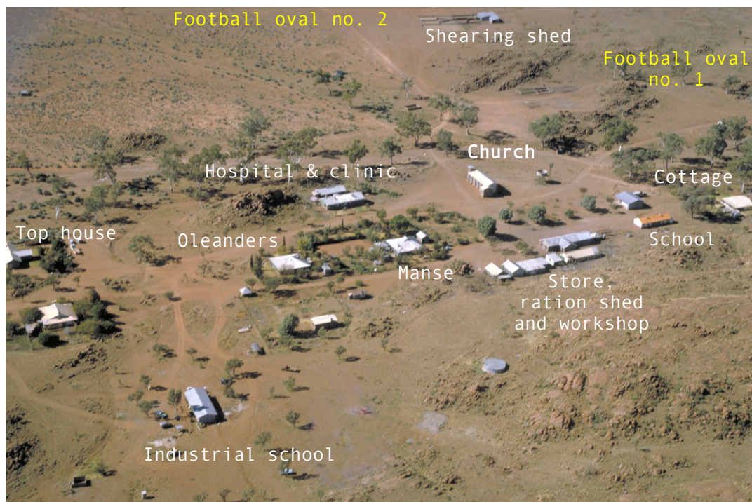
Figure 3. 1 Aerial view of mission from plane, 1967. Source: Aṛa Irititja, Allan Wilson Collection, Archive AI-0005951. Note the tennis court between the Manse and Oleanders. Constructed by Superintendent Bill Edwards, the surface of the court was made from hard, tightly compacted soil collected from ant mounds (Cameron, 2015).
