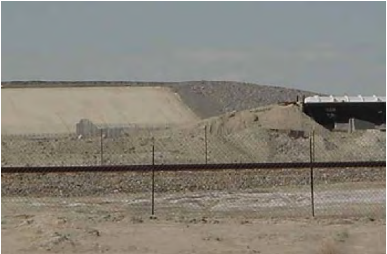
Fig. 2.1 LARW Waste Embankment Cell
