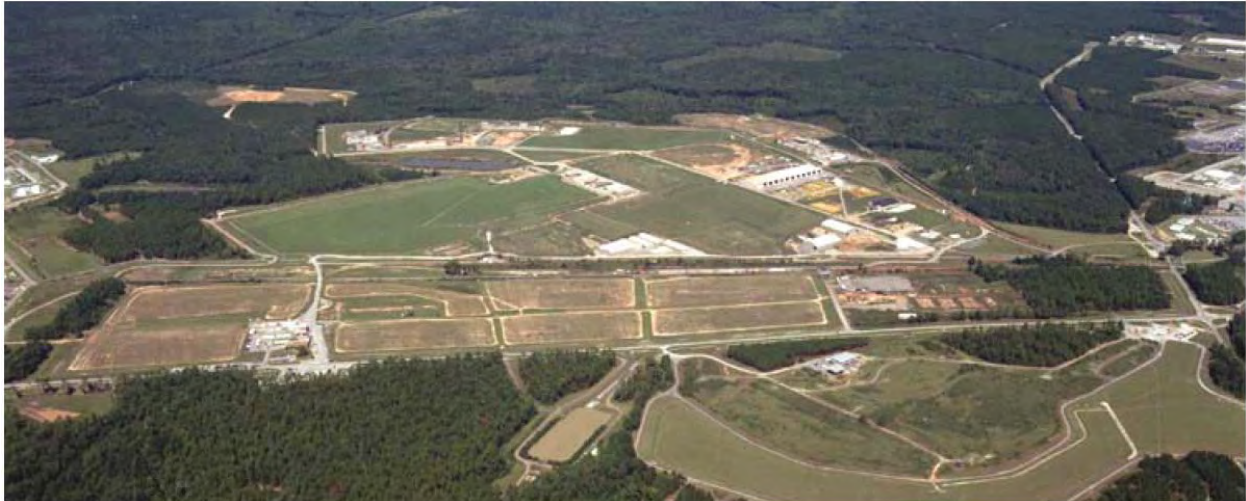
Figure 27: SRS plans to complete up to more than 70 additional waste sites in the next three years.
