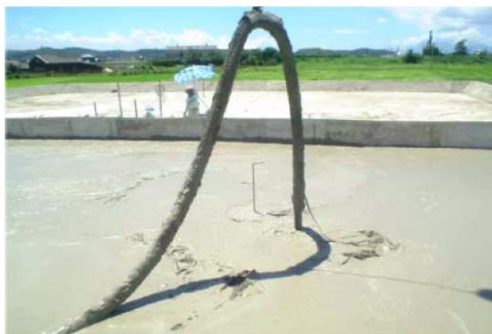
a. Embankment construction in progress
