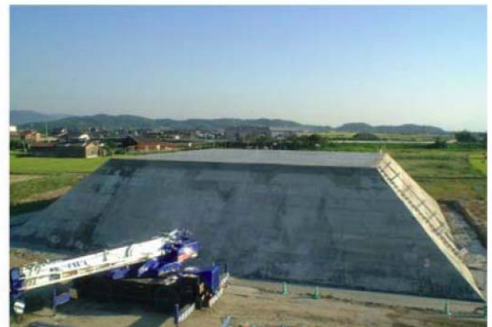
b. Completed embankment
