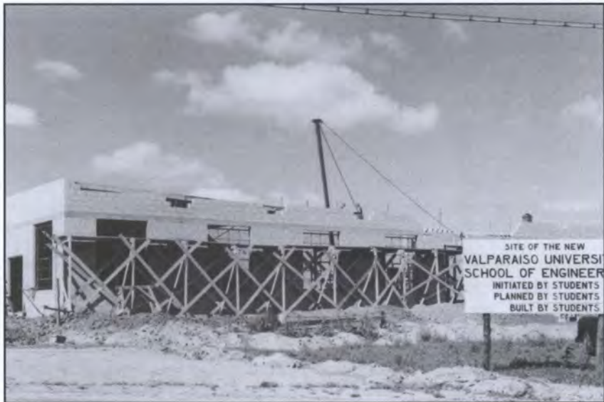
Under construction with the "historic" sign
