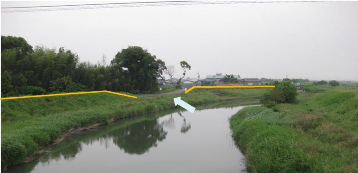
Figure 3.1 Overflow embankment of Jobaru River (Tsurunishi District, Kanzaki City, Saga Prefecture). (Ohgushi K., 2012)
