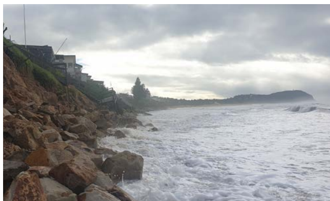
Storm surge exposed rocks and damaged infrastructure at Wamberal Beach, New South Wales, July 2020.
