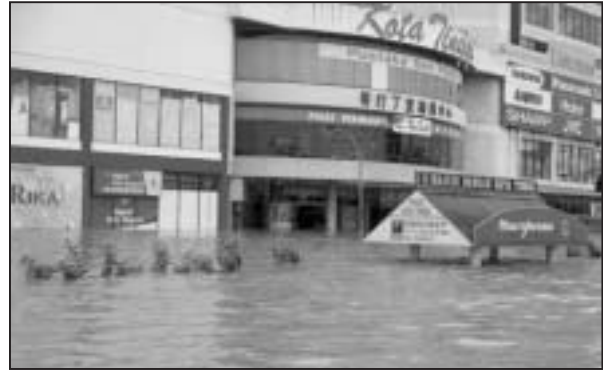
Fig. 2 Flood at Kota Tinggi town in January 2007
